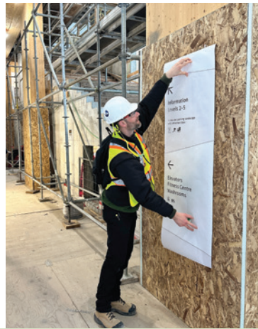
Both paper mock-ups and full-scale prototypes were used to verify sizing, placement, and architectural integration.
