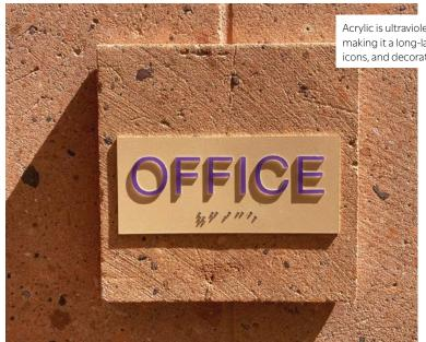
Acrylic is ultraviolet (UV)-stable and weatherable outdoors, making it a long-lasting material for compliant tactile letters, icons, and decorations.
