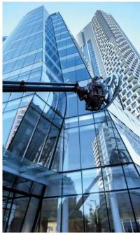
Keep your eyes on the sky as the weather can change in an instant, turning a routine lift into a high-risk situation. Strong winds don't just shift loads; they can make them feel heavier and harder to control. Lightning in the area is a clear sign to reassess whether it is safe to continue. Rain can quickly turn stable footing into an unpredictable hazard. Adaptability is key because, in this industry, the safest lift is the one that takes every element into account.
